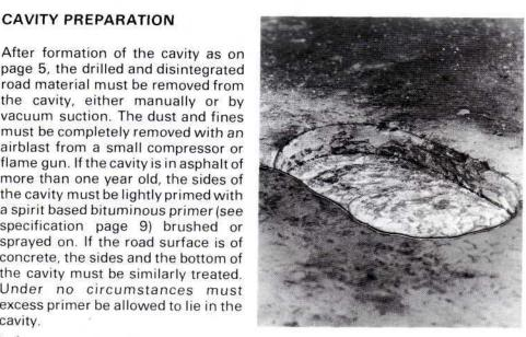
In frosty or wet conditions the cavity walls and base must be preheated by flame gun to dry off any dampness and to raise the temperature of surrounding road surface to a minimum of 5°C before applying the prime coat and before bedding and grouting the stud. Excess heat to the surrounding asphalt should however be avoided, as this will damage the material and failure of the installation may result
