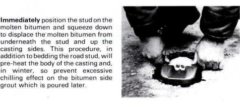
Check the overall height of the stud with the aid of the height gauge. The gauge must be rested on the casting reflector recess platform and should show a gap between the bottom of the gauge and the road surface of between 0 and 3mm (see page 3).
