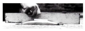
The road stud (either type) must be paved so that, with the height gauge resting on the casting flanges (as shown in the photograph) the ends of the gauge should also be in contact with or just clear of the road surface.
