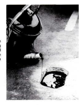
molten bitumen and squeeze down to displace the molten bitumen from underneath the stud and up the casting sides. This procedure, in addition to bedding the road stud, will pre-heat the body of the casting and, in winter, so prevent excessive chilling effect on the bitumen side grout which is poured later.
